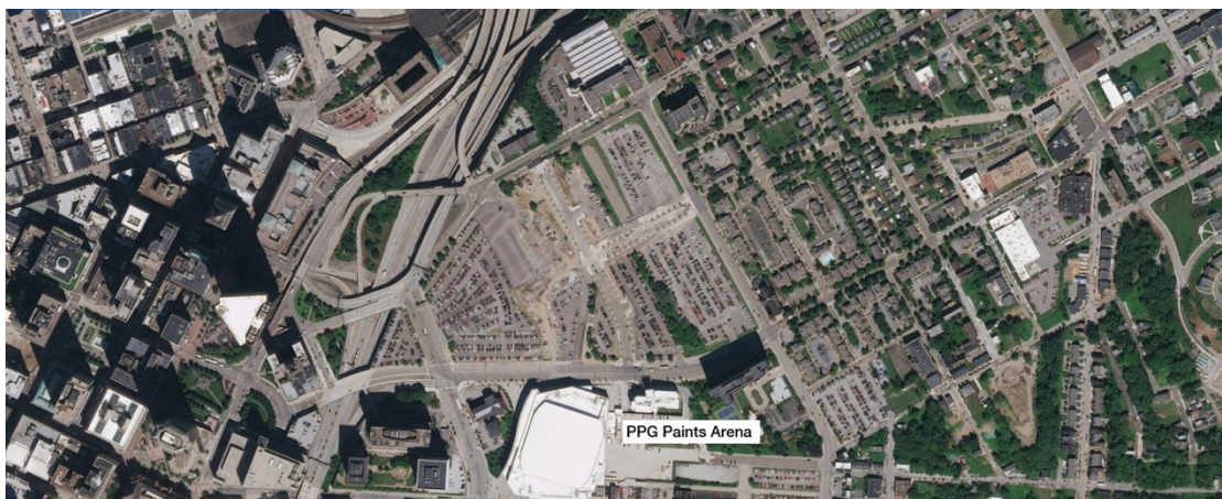
Figure 5.6 Aerial view of Lower Hill featuring demolished Civic Arena and subsequent parking lots
