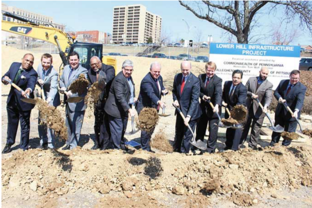
A NEW DAY DAWNS—Federal, state and local partners break ground for the first phase of the $440 million project to redevelop the lower Hill District and to rebuild the Hill and beyond. (Photo by J.L. Martello)
