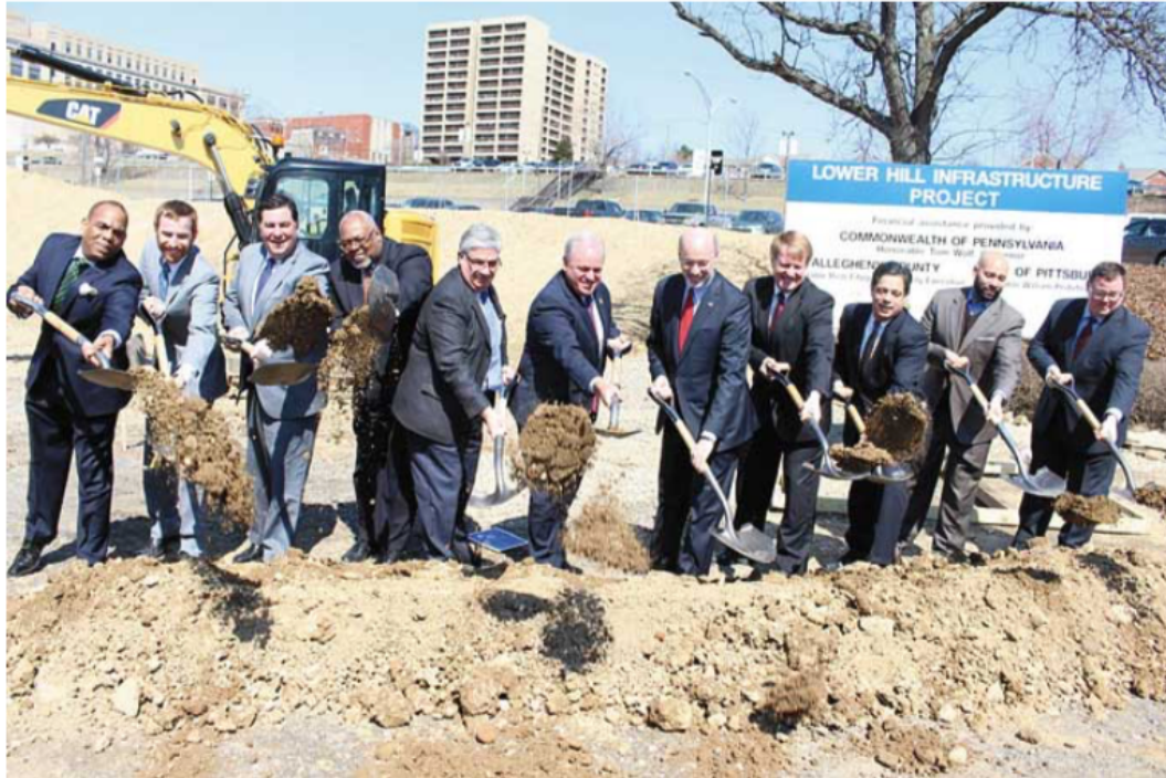
A NEW DAY DAWNS—Federal, state and local partners break ground for the first phase of the $440 million project to redevelop the lower Hill District and to rebuild the Hill and beyond. (Photo by J.L. Martello)
