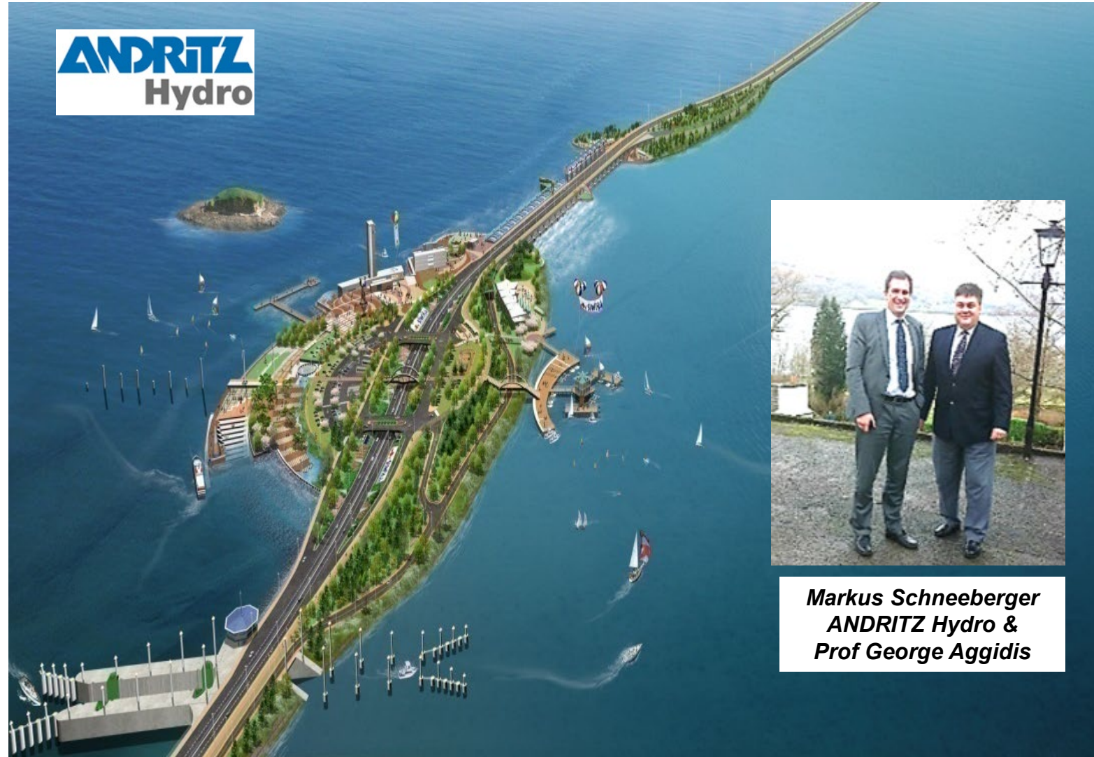
Sihwa, South Korea tidal power plant 2011
