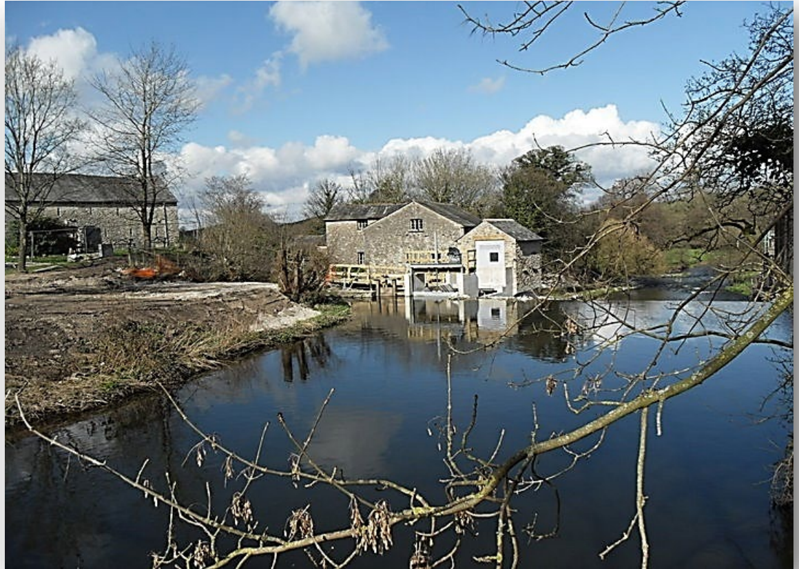
After the completion of the Low Head Hydro Plant
