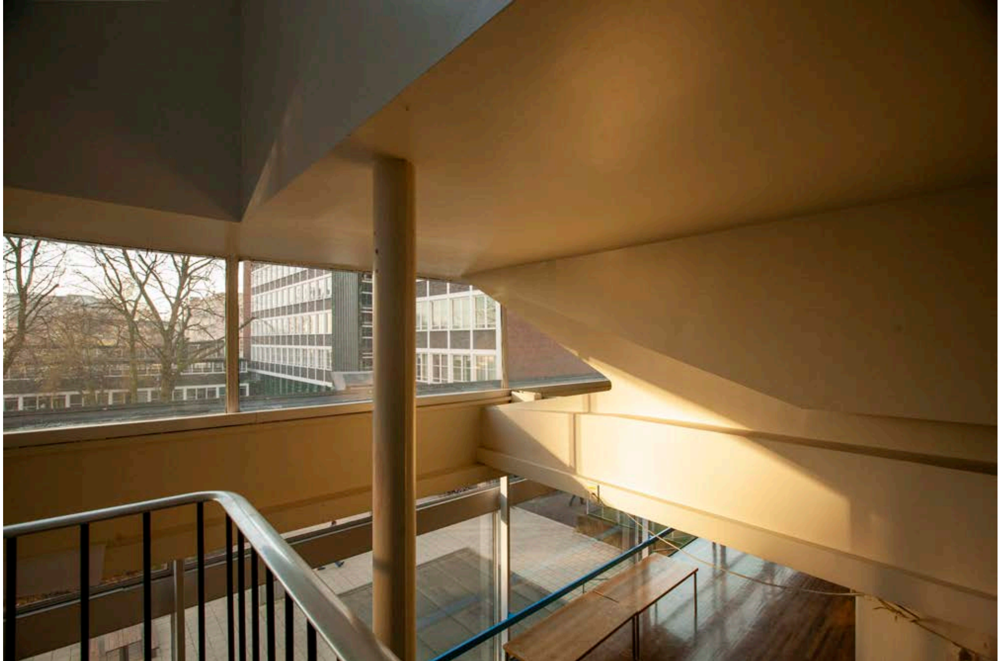
Renold Building, rebated birds mouth beam, post-stressed, pre-tensioned.
