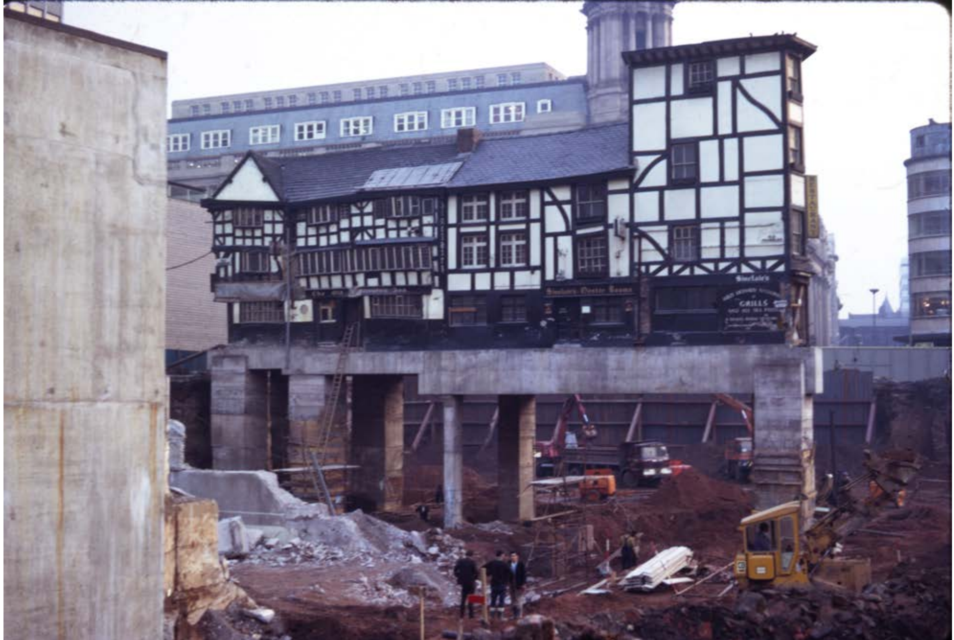
The raising of the Old Wellington Inn and Sinclair's Oyster Bar.
