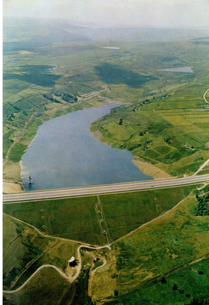
Scammonden dam and reservoir. Aerial view from the north c.1971.
