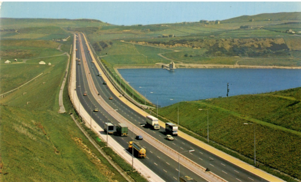
M62 Motorway and Scammonden Dam, Huddersfield
