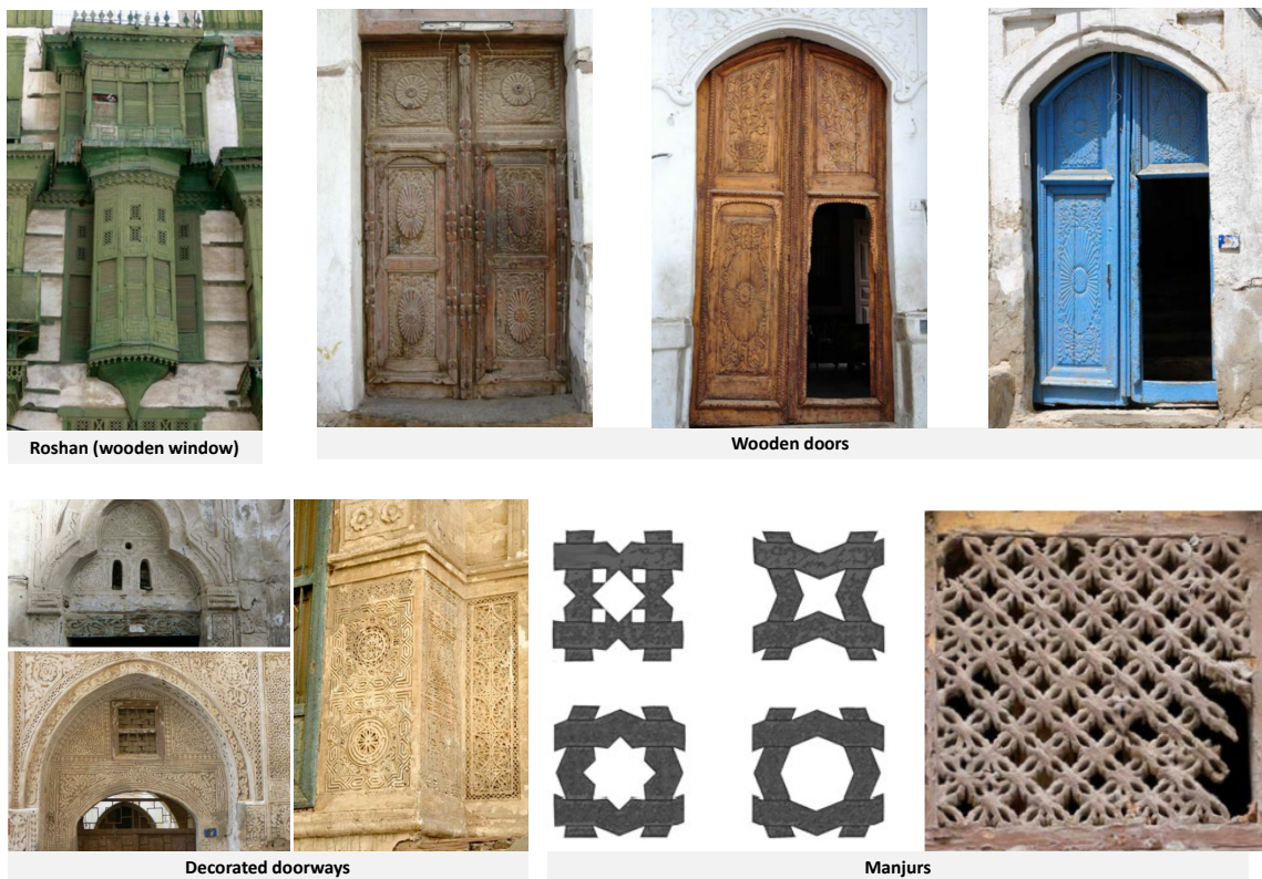
Figure 4. 14: Examples of Roshan (Wooden window), wooden doors, decorated doorways, and Manjurs in Jeddah buildings. (Saudi Commission for Tourism and Antiquities, 2013, pp.52-58)
