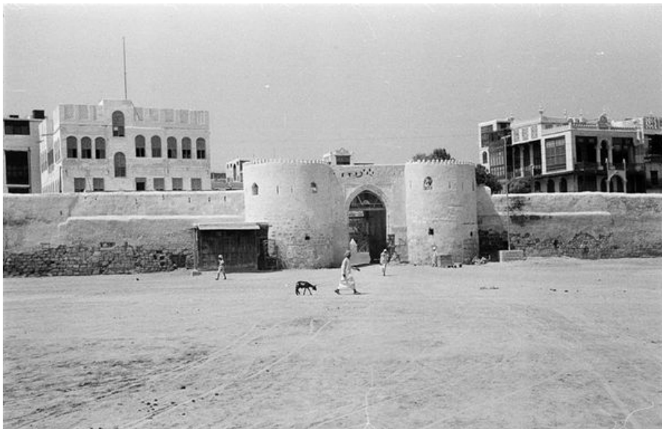
Figure 4. 19: The Madina Gate in 1918 at the top, and the bottom before demolishing the wall, the picture from 1945 by the globetrotter Wilfrid Thesiger. (Abu Alama, 2010; The Pitt Rivers Museum, 2012)
