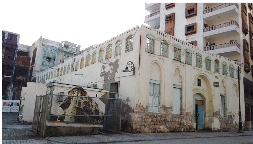
Figure 5. 35: Electric stations and metal fencing located beside and backside the building. (Author, 2021)
