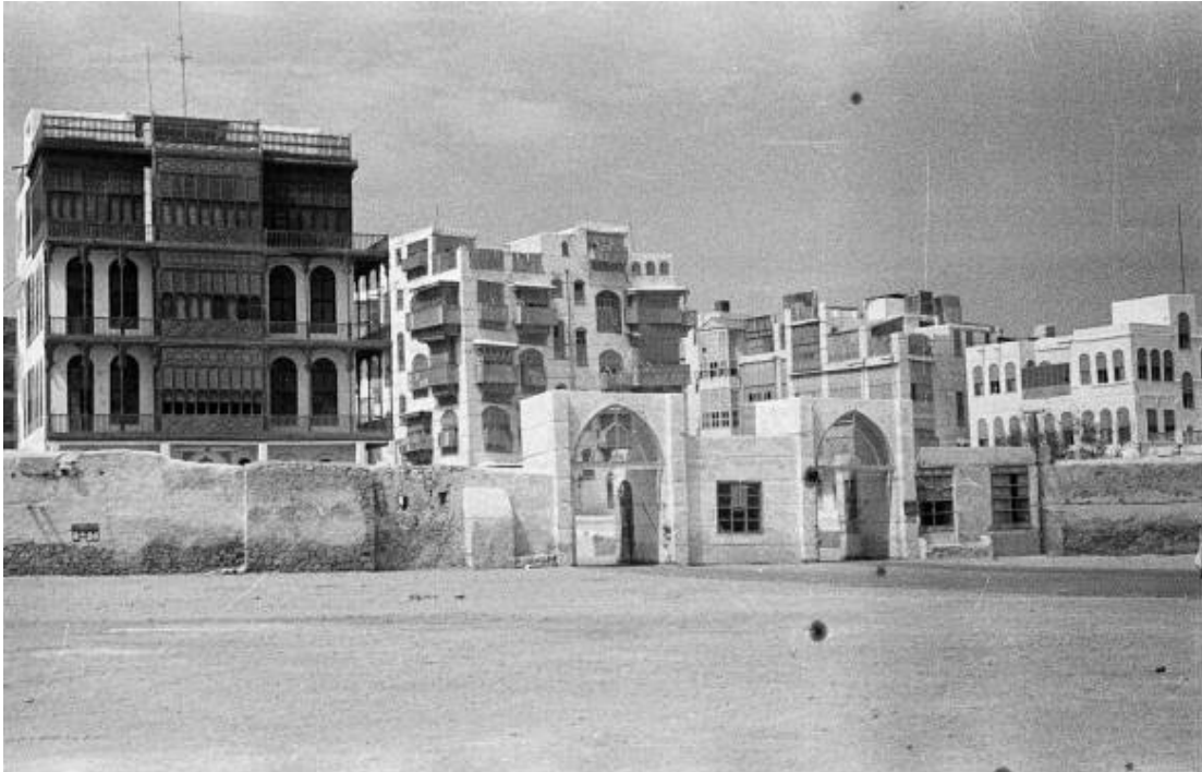
Figure 4. 21: The Jadid Gate in 1945 AD before demolishing the wall in 1947 AD. Source: Dr. Zaher Othman, Photograph by: Wilfrid Thesiger. (Bakr, 2014; Othman, 2019)
