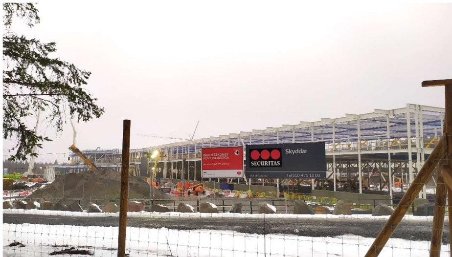
Figure 32. Erecting Facebook’s fourth data centre building in snow, Luleå, October 2020.
