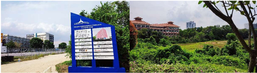
Figure 28. Cyberjaya’s centre. These particular plots may be reserved for future builds, but the entire area is quite spacious. In other words, it would be easy to place dehydration plants here, as well as to gain access to the sites.
