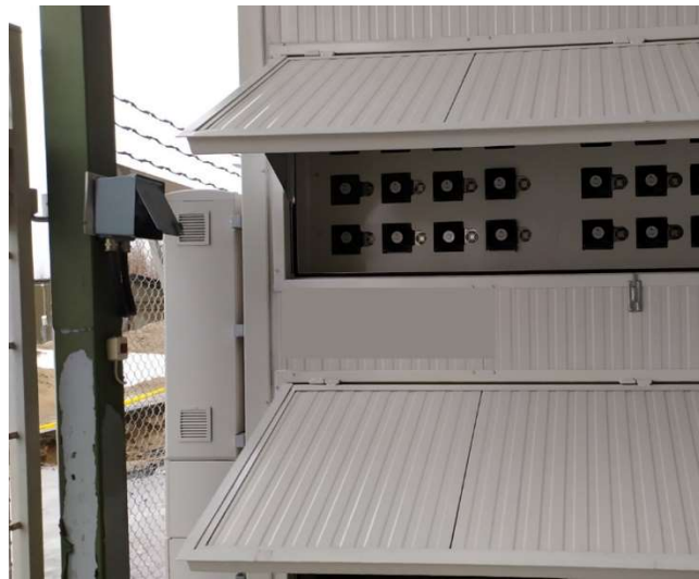
Figure 12. Crypto mining in October 2020 using graphical processing units (GPUs) in the vicinity to Luleå, Sweden. On this latitude, and with unpolluted air, servers can take advantage of free cooling (note the snow in the background). The photo shows parts of a system of 500 kilowatts of bitcoin mining in progress.
